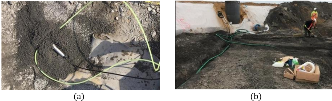
Figure 3-8: (a) Hydraulic transmitters installed at level of the RI, (b) wiring to the acquisition units.
