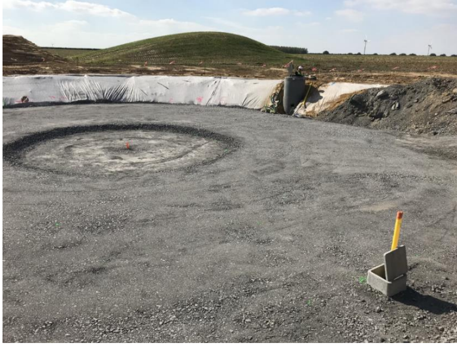
Figure 3-11: Position of the inclinometer.
